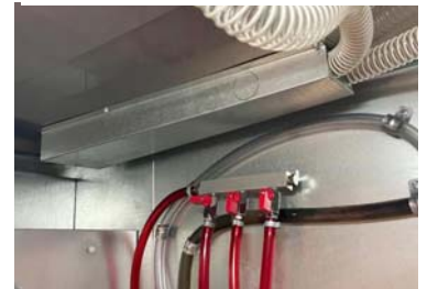
Air Channel Conversion Kit Convert Back Bar to Direct Draw Dispenser
